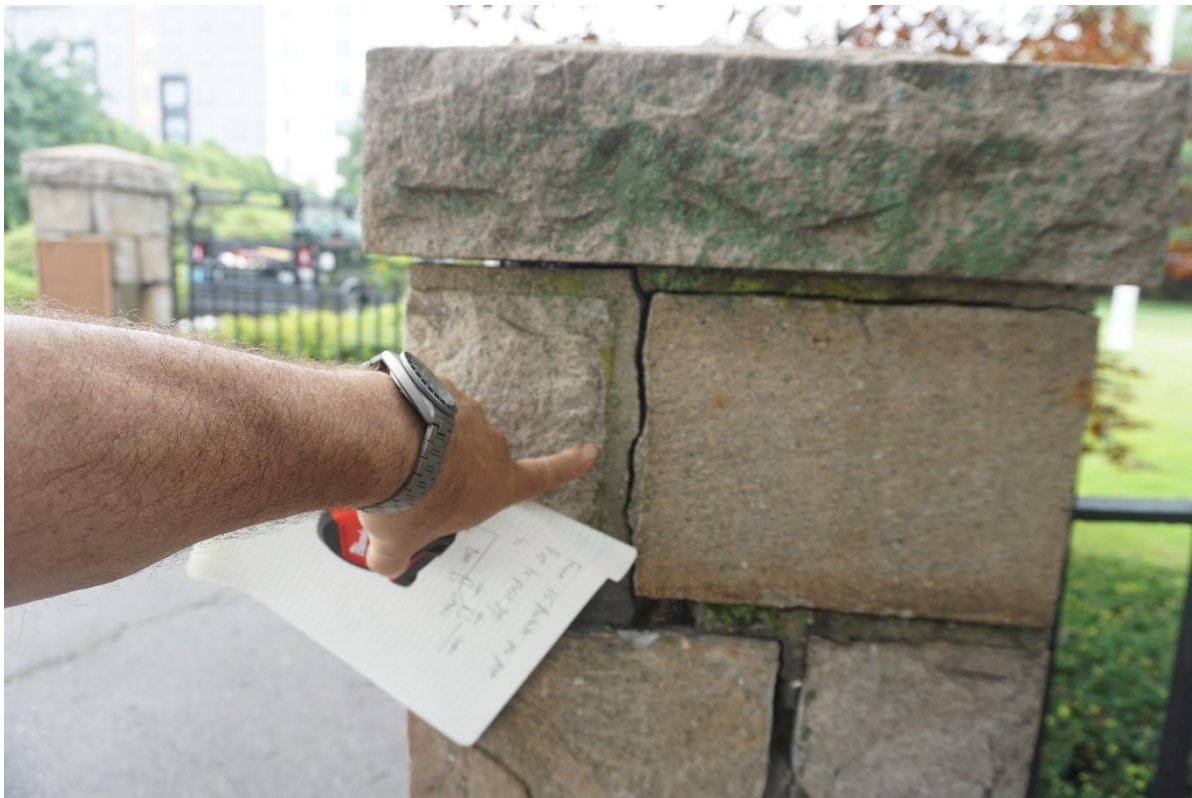
Degraded Mortar on Post
